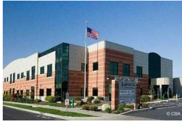
Iron Bridge — Building III 42,240 SF | $200/SF $8,460,368 05/08/23 Built: 2008
